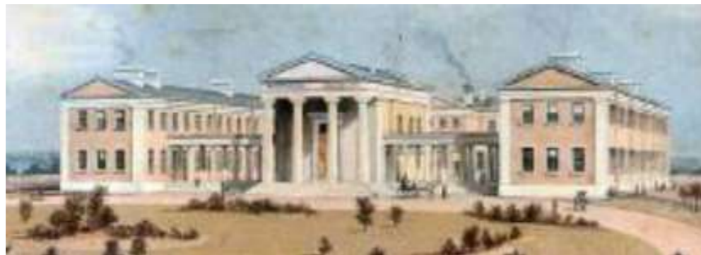
Figure 2 – Original Portico Building
